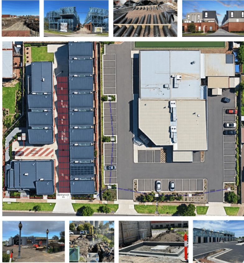
Townhouse drainage works (top) and carpark drainage works (bottom), either side of the aerial overview of the completed stormwater strategy — carpark rain gardens (right) and the townhouse raintank/OSD network beneath the central driveway (left), Talmage Street.
